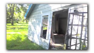
• There are signs of excessive wood destroying insect damaged and possible infestation at the Left and Back exterior walls. There appears to be around 1/3 wall studs damaged by wood destroying insect infestation. Any damaged wood should be repaired and properly reinforced or be replaced. Consult a pest control company to evaluate and eliminate potential wood destroying insect infestation. Also consult a framing contractor to make any needed repairs.
