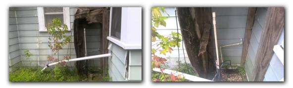
Note: The gas supply was disconnected at the time of the inspection. The gas meter was not present leaving the pipe cut.
