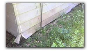
• There is wood rot observed at the left side and back wall siding and trim boards. Any damaged wood should be repaired and properly sealed to limit further deterioration or be replaced.
