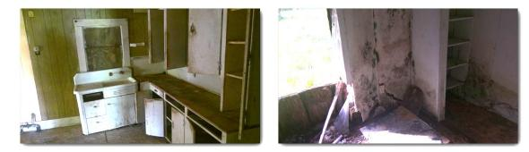
• There are moisture stains observed at the living area, kitchen, bath and right side Bedroom wall. When tested these stains did appear current. Any moisture stains should be painted and repaired to limit organic growth. The damage dry wall should be repaired.
