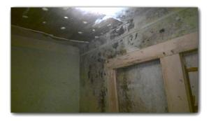
• There are signs of wood destroying insect damage observed at the Bedroom, Utility Room, Kitchen, Bathroom, Entry walls and wood trim. Any insect damage should be repaired and properly finished to match.
