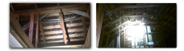
There are sections of missing insulation observed at the attic throughout. There should be R-30 insulation present. Any missing inspection should be replaced to increase energy efficiency.
