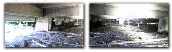
The floor decking is observed sloping more than 1" in 4' at both the shop and house interior floors throughout. This deflection does appear to be excessive enough to warrant possible repair. Consult a foundation leveling company to check the floor system and make any needed repairs.
