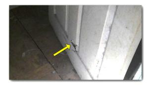
• The kitchen/hall room door frame and trim is split and damaged. The left side exterior door and frame are damaged and partially missing. The damaged door frame and trim should be replaced.
